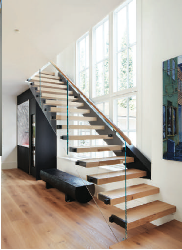
TREAD LIGHTLY: Dark, heavy stairs are replaced with "floating" treads and glass to allow maximum light to enter the home.
